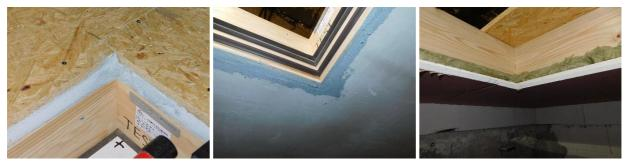
Around the perimeter of opening for the shutter, mineral rock wool of type Toprock Super, 30 mm thick, with bulk density of 40 kg/m³ (manufacturer: Rockwool) in width of 200 mm is applied.
